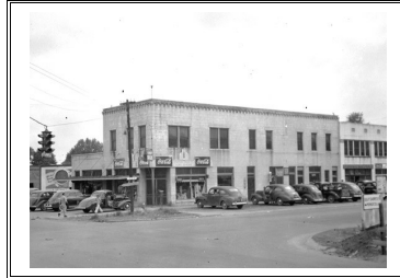
Holmes Hospital upstairs
